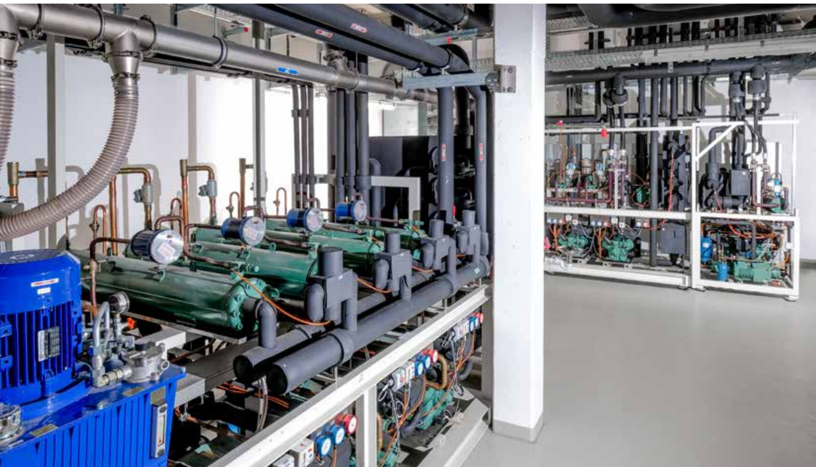
Engineering area with refrigeration system for several freeze dryers
